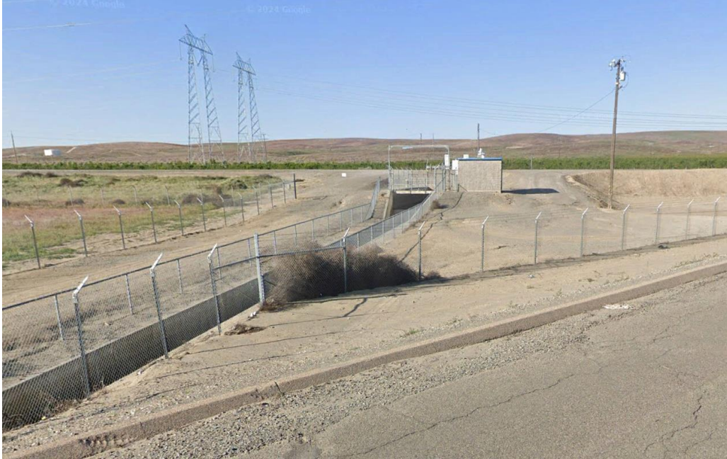
California Aqueduct Intertie
