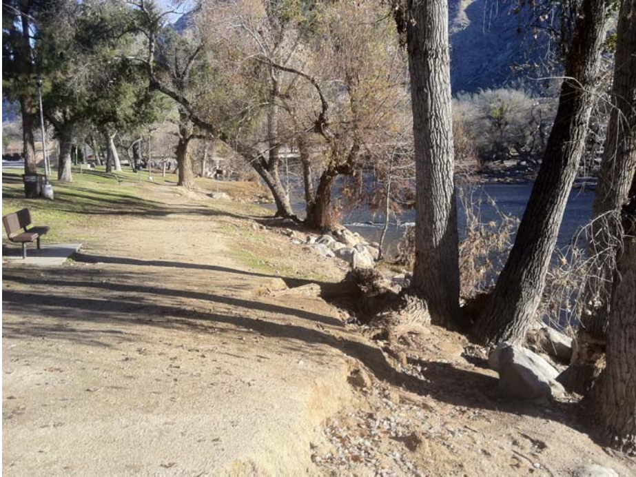
Figure 9: Erosion exacerbated by insufficient stabilization
