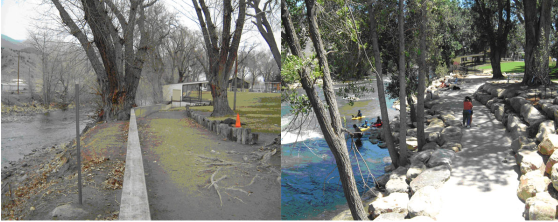
Figure 16. Before and after example of bank terracing and trail improvements in Salida, CO
