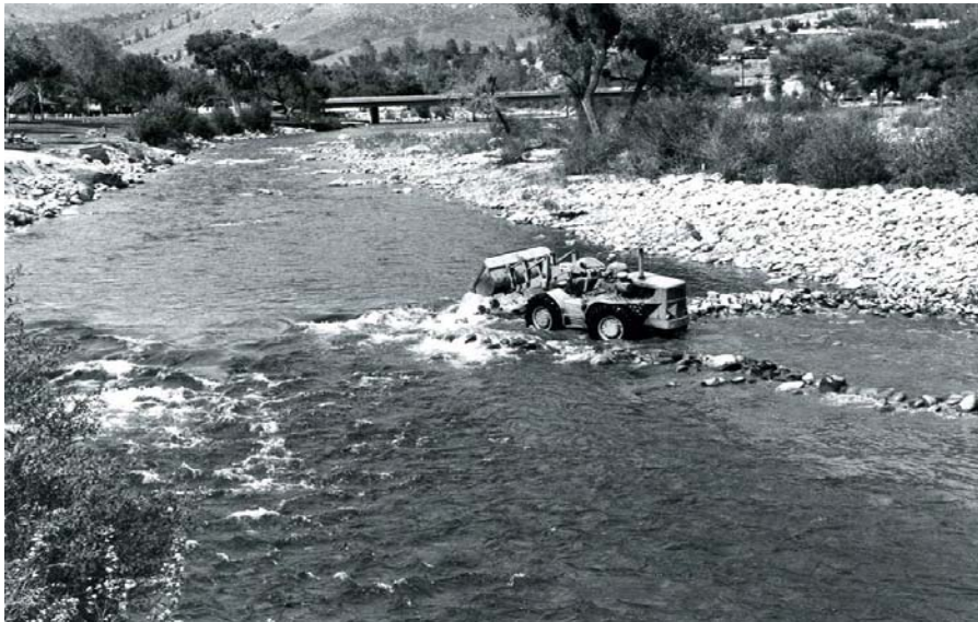
Figure 2: Construction photo of the original bank barbs
