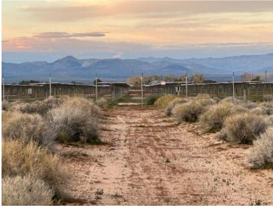
Photo 4-6.1: RB Inyokern Solar Project (Fence north of Project site)
