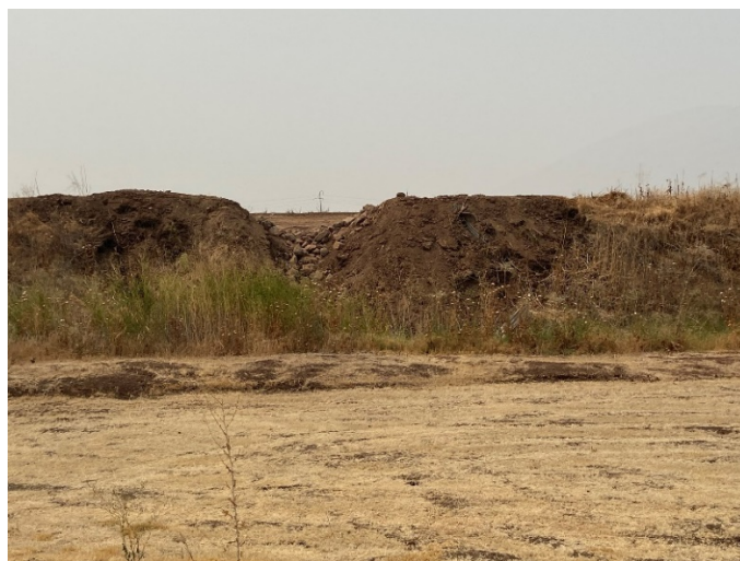
Embankment was cut out and armored with rock to allow runoff and minimize erosion.
