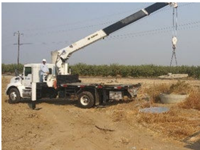
Delano Staff removing a manhole cover
