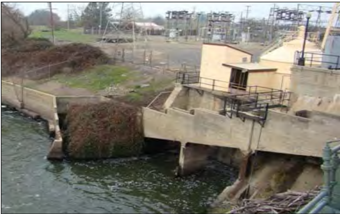
Figures 1 and 2: Two views of the fish ladder from the top of PG&E's Merced Falls Dam on the Merced River. Photos taken February 2, 2010.
