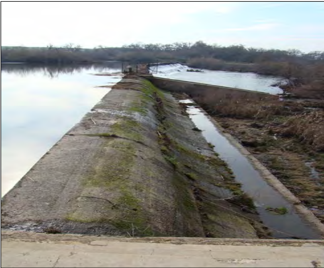
Figure 4. View of the Crocker-Huffman Dam from the river right bank. In the foreground is the ogee spillway. Beyond that is the fish ladder, followed by the primary dam crest.
