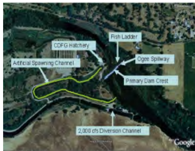
13 14 15 Figure 2: Overview of Crocker-Huffman Dam complex 16 McKinnon Declaration WAC 000017
