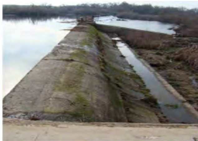
13 14 Figure 3: View of the Crocker-Huffman Dam from the river right bank. 15 In the foreground is the ogee spillway. Beyond that is the fish ladder, followed by the 16 primary dam crest.
