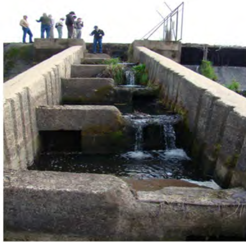
Figure 5. View looking upstream at the fish ladder at the Crocker-Huffman Dam. One of the original orifices is visible. All weirs have been notched to the river-left side (to the right side of the photo).
