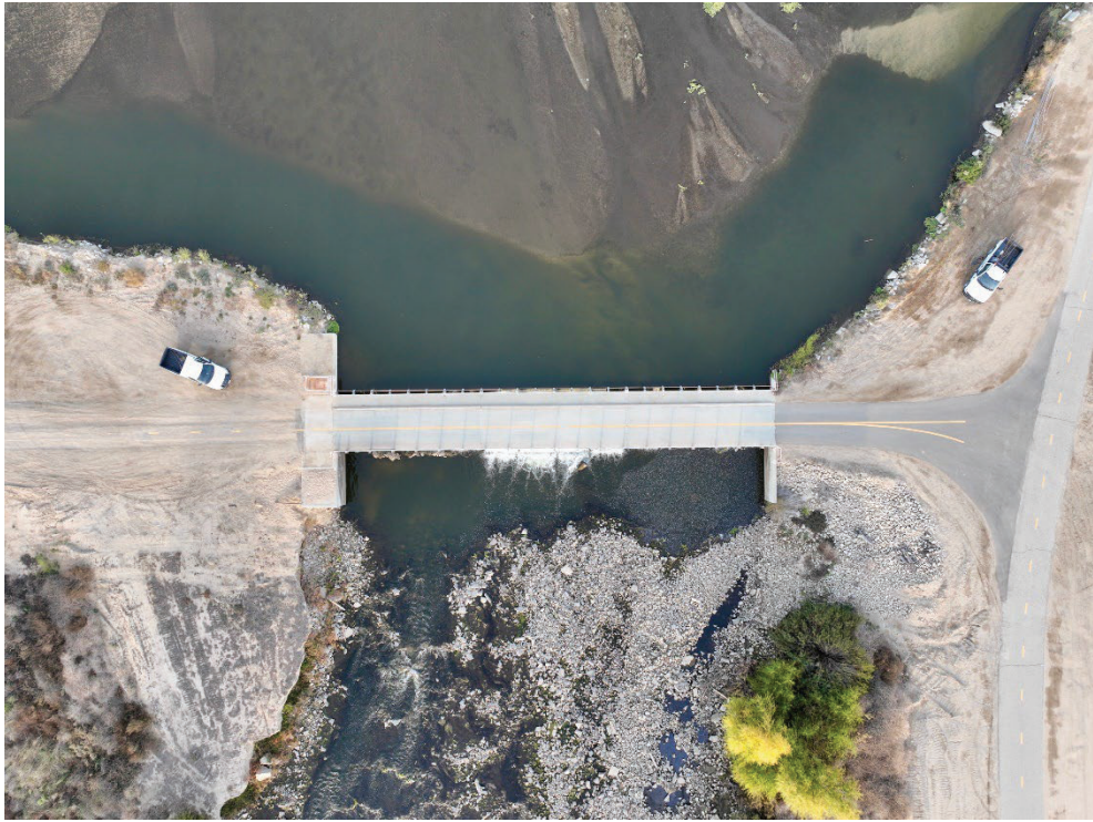
Top of Weir
