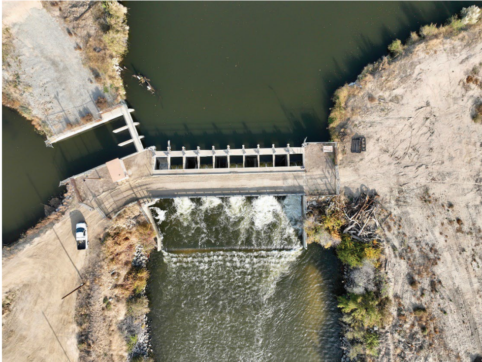
Top of Weir
