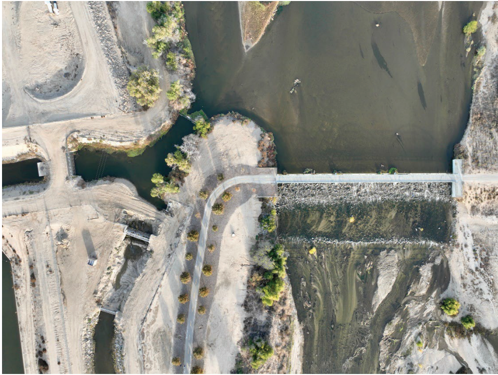
Top of Weir
