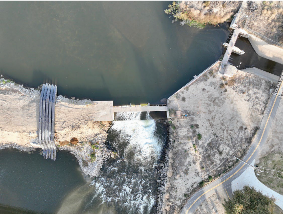
Top of Weir
