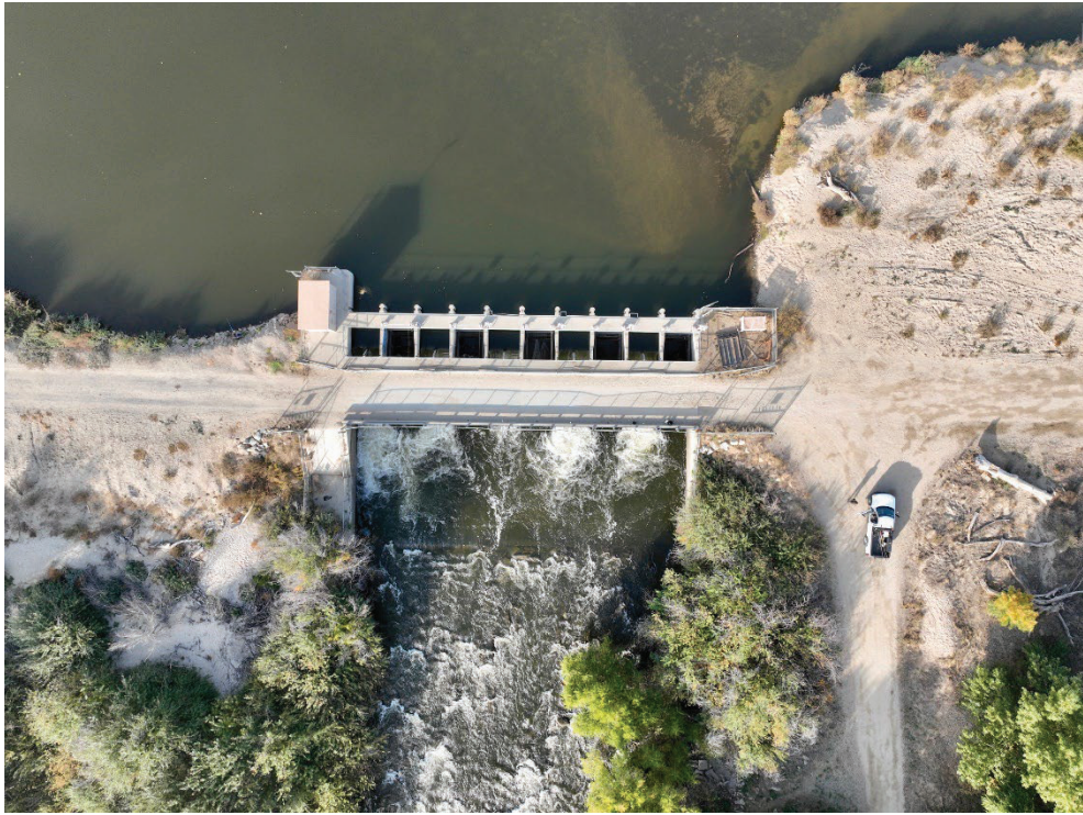
Top of Weir
