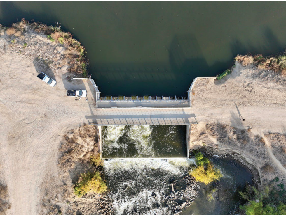
Top of Weir
