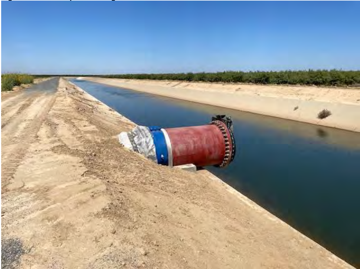
Figure 2-4. Example Discharge Outfall.
