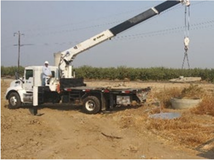
Delano Staff removing a manhole cover
